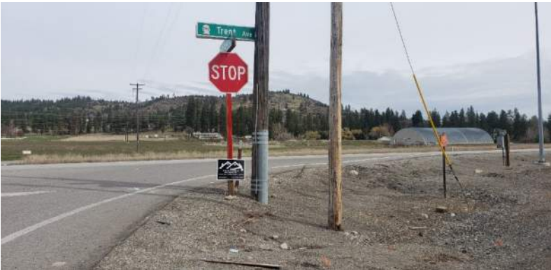
IMAGE 14: McKinzie Rd at Trent Ave, stop bar worn, broken reflectors
