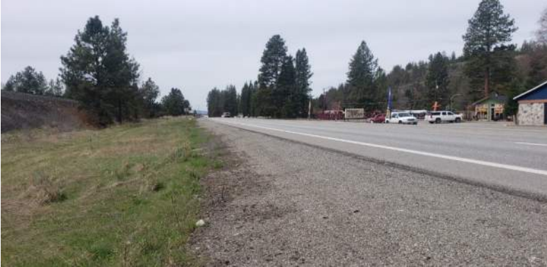
IMAGE 19: Trent Ave south shoulder at Starr Rd, space to add right turn lane
