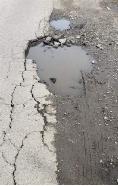
IMAGE 22: Starr Rd northbound, shoulder pavement
