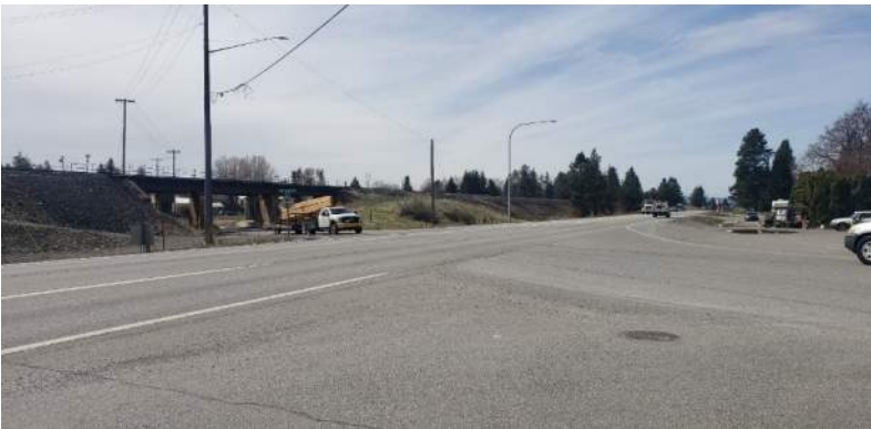
IMAGE 25: Trent and Starr intersection offset, looking SW
