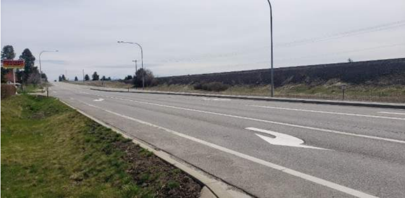
IMAGE 26: Trent Ave westbound right turn lane and swale behind curb
