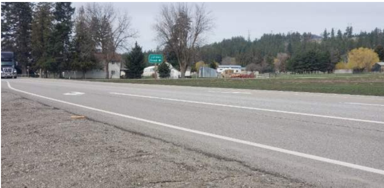
IMAGE 12: Trent Ave eastbound right turn lane at McKinzie Rd
