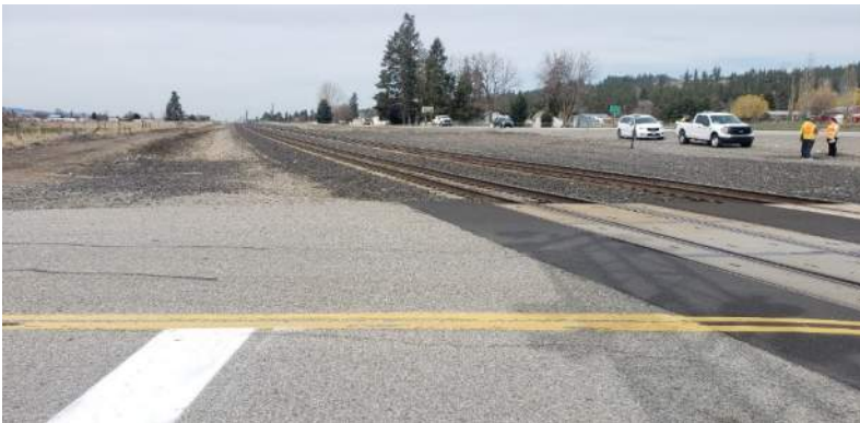
IMAGE 11: McKinzie Rd rail crossing looking west
