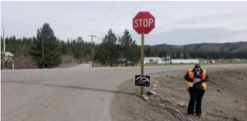
IMAGE 6: Harvard Rd northbound, worn striping, missing stop bar, stop sign bent
