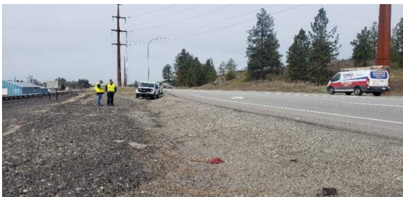
IMAGE 2: Trent Ave shoulder at Harvard Rd, looking west at right turn lane
