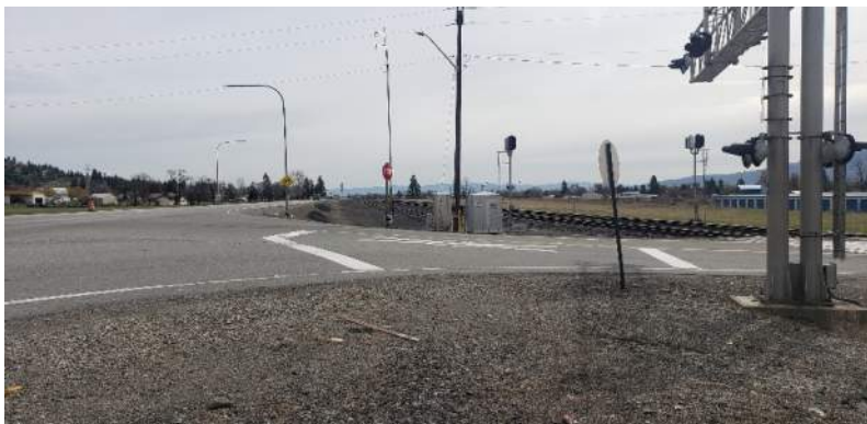
IMAGE 3: Trent Ave Eastbound at Harvard Rd, broken reflector
