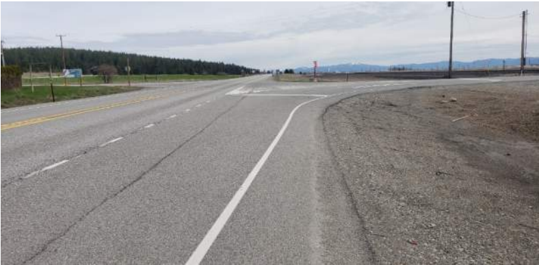
IMAGE 30: Trent Ave eastbound right turn lane at Idaho Rd
