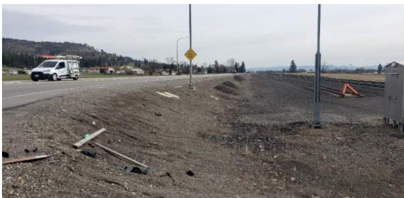
IMAGE 4: Trent Ave EB shoulder at Harvard Rd, debris, broken reflectors
