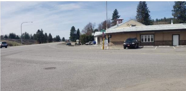
IMAGE 28: Trent Ave westbound at Starr Rd, vehicles can cut through parking lot to get around stop sign
