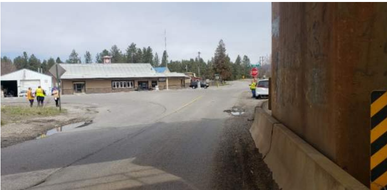
IMAGE 21: Starr Rd northbound visibility under rail bridge
