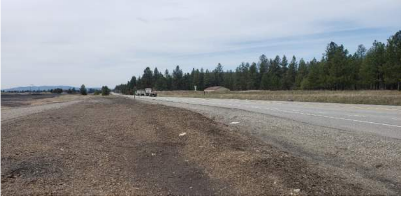
IMAGE 29: Trent Ave south shoulder at Idaho Rd looking west
